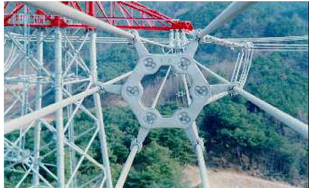
6 bundle conductor and spacer
