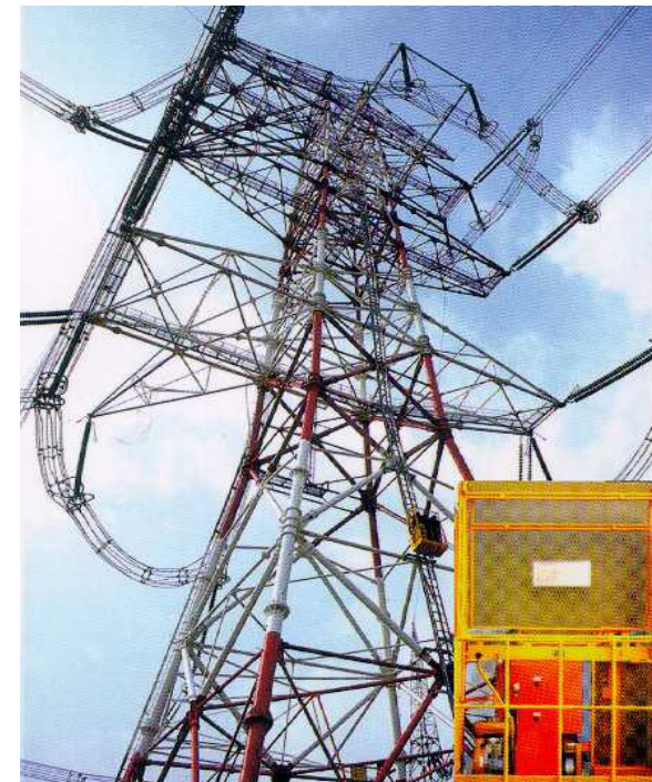
Lift for tower and its rail
