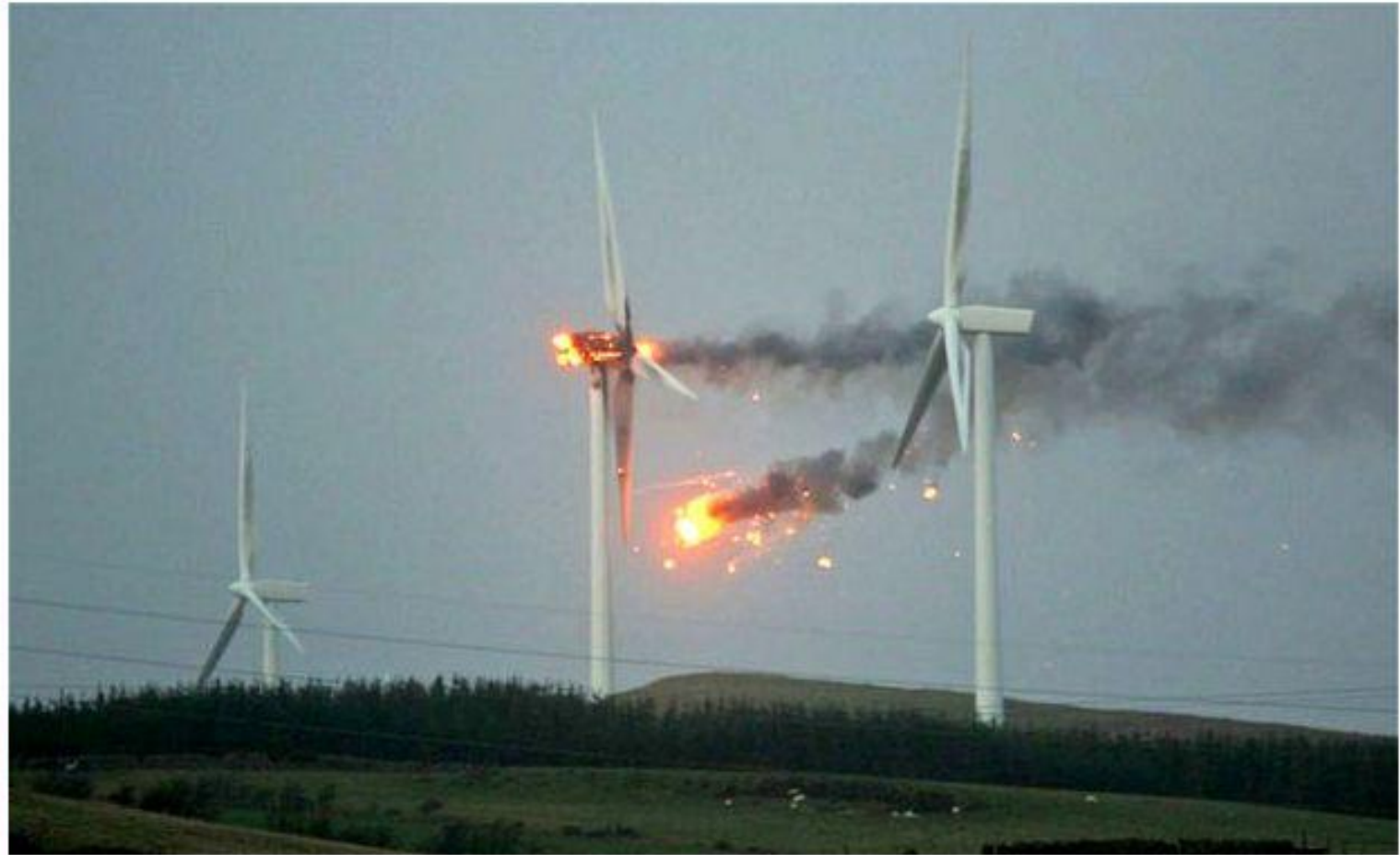
A £2 million, 100 metre tall wind turbine catches fire in hurricane-force winds at Ardrossan, North Ayrshire, Scotland. The wind turbine was spinning so fast it caught fire. The engine of the giant turbine went up in flames and its blades were blackened by smoke. The turbine was one of 15 set up on hills overlooking the Scottish coast, built to supply green electricity to 20,000 homes.
