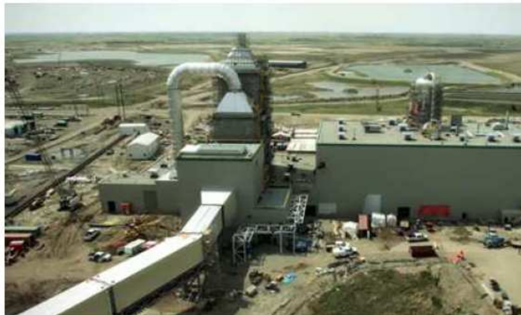
Boundary Dam CCS power plant in Canada. Photograph: SaskPowerCCS
