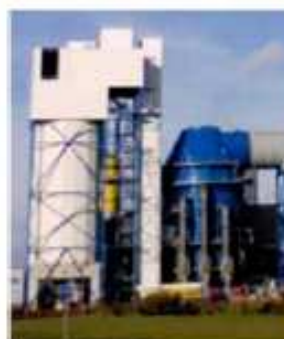
Alstom Wet Flue Gas Desulfurization
